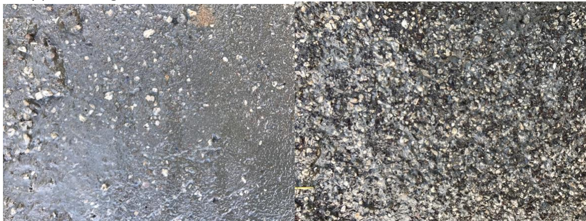
Eroded - with gentle water blasting
